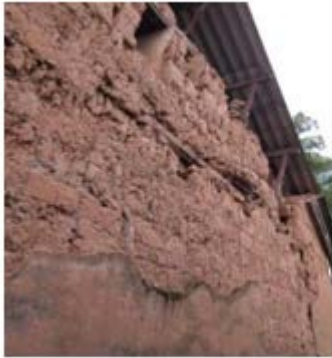
Fig 1. rammed earth wall with weathered cracks Fig 2. brick wall after demolition
